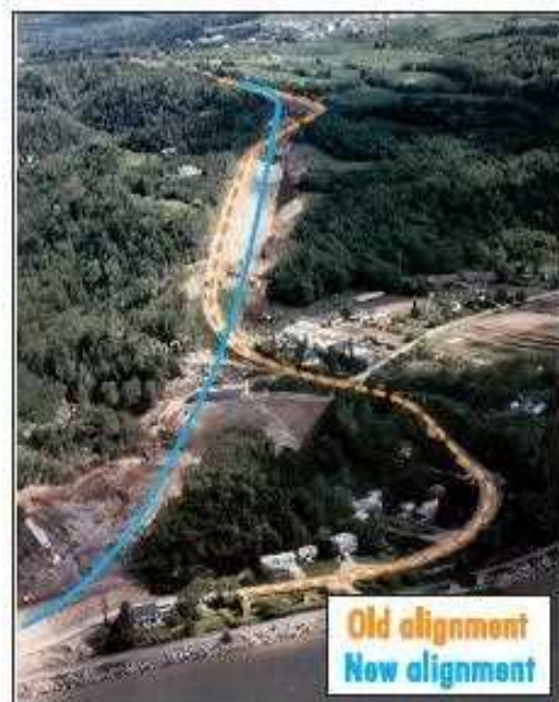
Alignment modification to eliminate a sharp curve at the bottom of a steep grade
